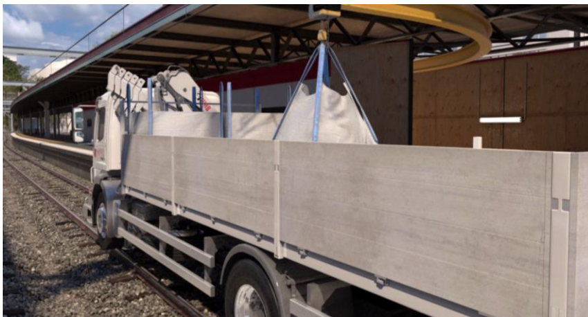
Figure 3.2: Eastern Concourse Construction – Spoil Removal
