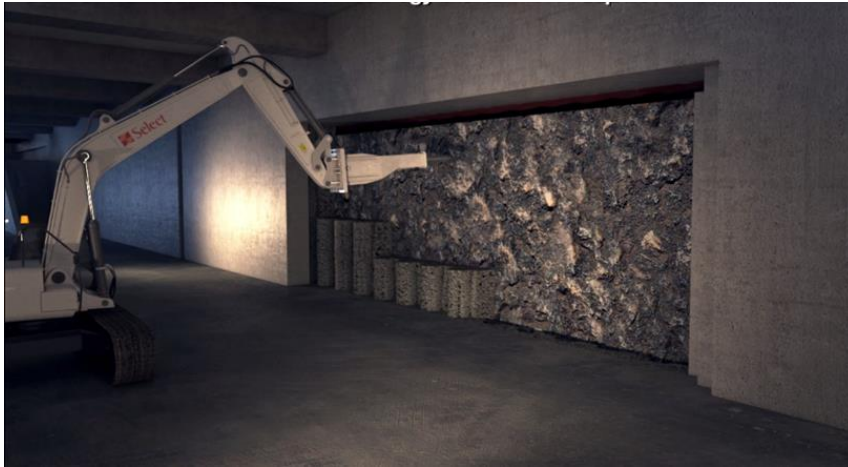
Figure 3.3: Eastern Concourse Construction – Mining
