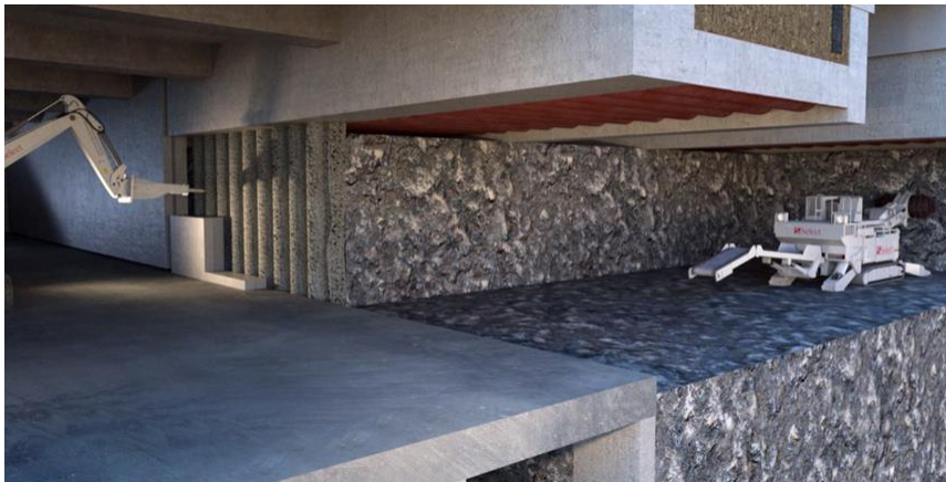
Figure 3.4: Eastern Concourse Construction – Road Header Mining
