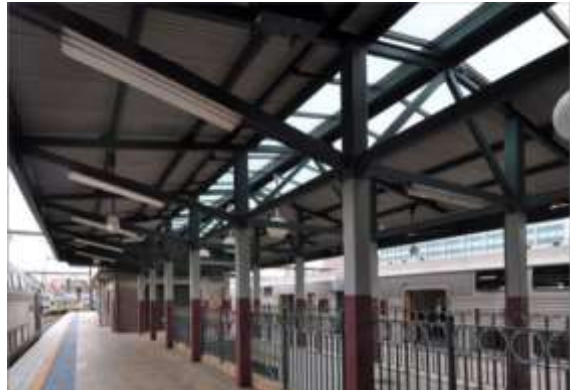
Figure 3: Typical awning extension on the Sydney Terminal platforms and extant balustrading (Source: Rappoport, 2013).
