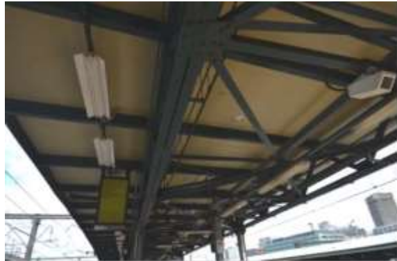
Figure 5: The steel trusses and reinforced concrete awning along the platforms (Source: Rappoport, 2013).
