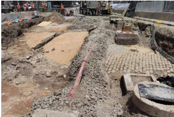
Figure 40: View (left to right) of curved tram track, concrete road base, and basalt cobblestone surface
