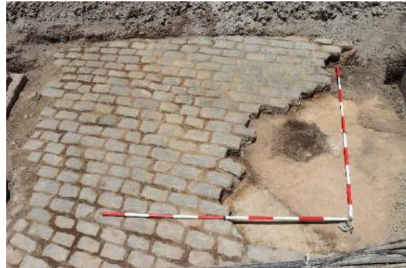
Figure 41: Detail of basalt cobblestone surface (left) showing concrete road base (right)
