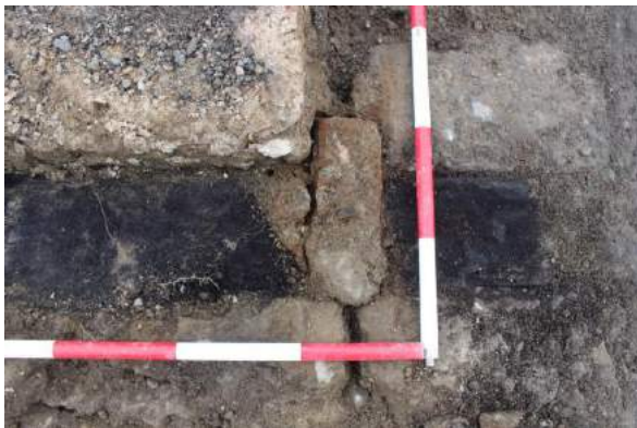
Figure 30: Detail shot of wooden sleeper and metal tram track
