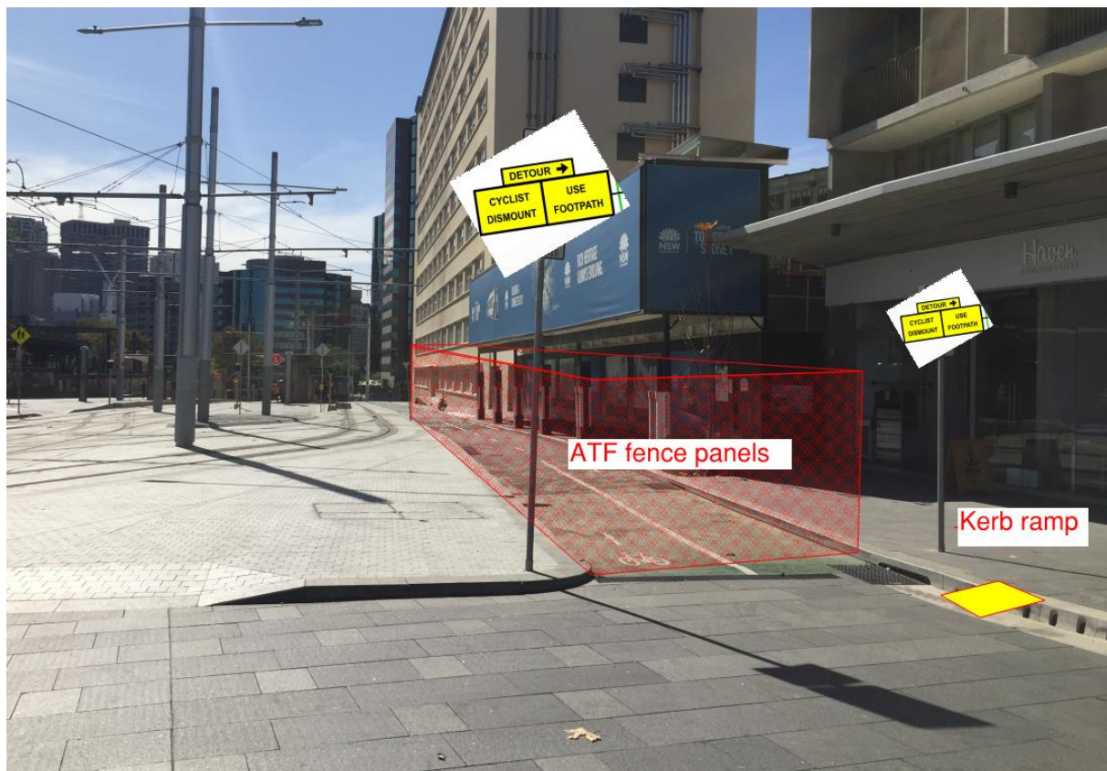
Figure six – Site photo showing location of site establishment for works in cycle lane
