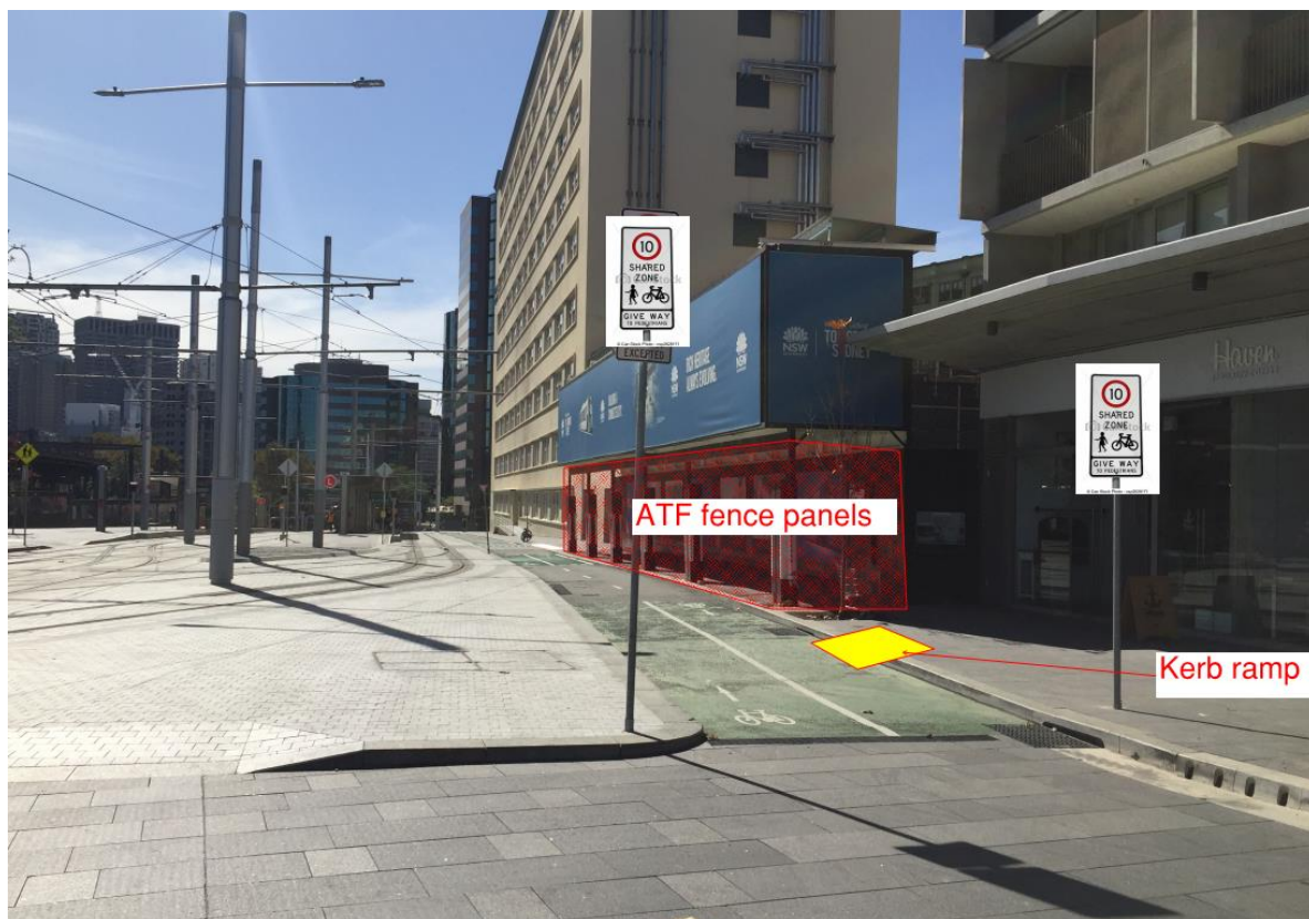
Figure four – Site photo showing location of site establishment for works in footpath
